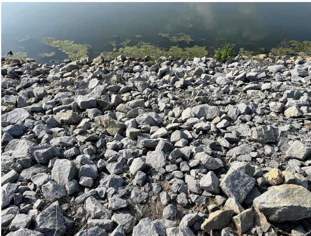
Figure A2. North Interior Slope of Pump Back Pond #2; 6/30/2023
