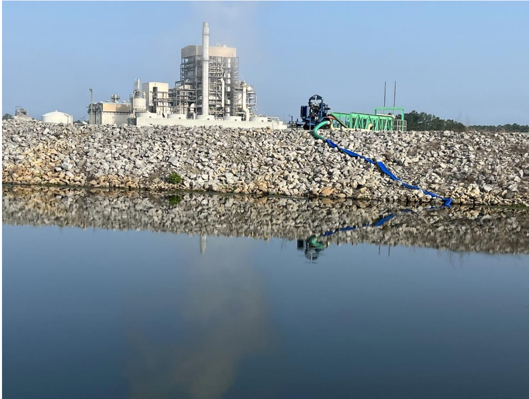
Figure A1. North Interior Slope of Pump Back Pond #2; 6/30/2023
